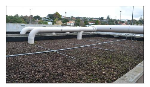
Figure 1 – Biofilter at Pump Station 64
